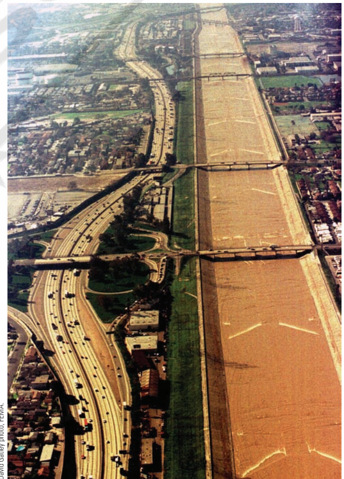
► FIGURE 12-16. The Los Angeles River runs through a straight section of concrete channel with angled energy dissipation structures.
