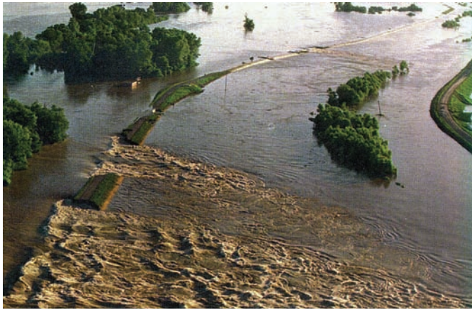
► FIGURE 12-7. In the breach of this levee during the 1993 flood on the Mississippi, the river (on the left) spills through two breaches to cover the floodplain (right). A second levee at the right edge of the photo provides temporary relief.
