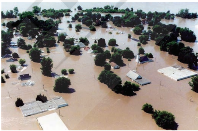
► FIGURE 12-9. The 1993 flood left a large number of homes deeply submerged in floodwaters for an extended period of time.
