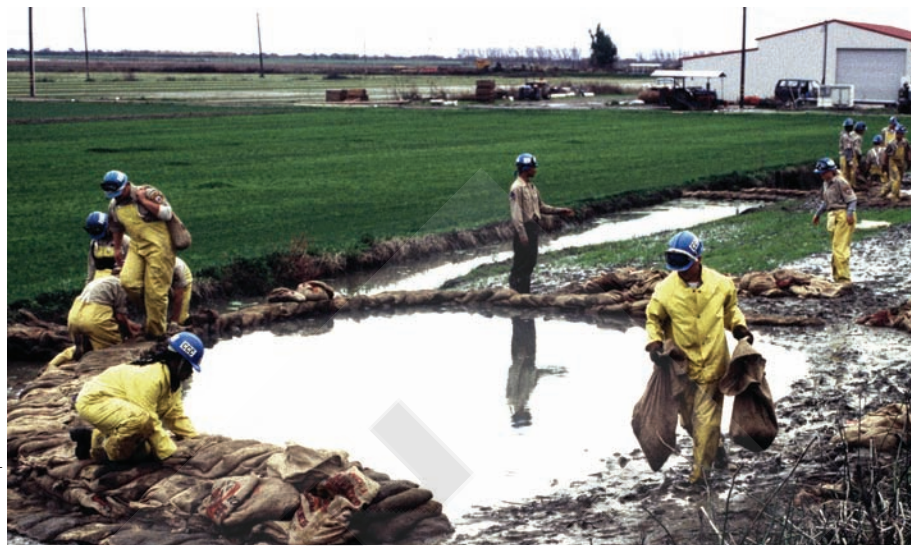
► FIGURE 12-4. A California Conservation Corps crew places sandbags around sand boils at the Sacramento River, at north Andrus Island, in the delta area southwest of Sacramento on January 4, 1997.
