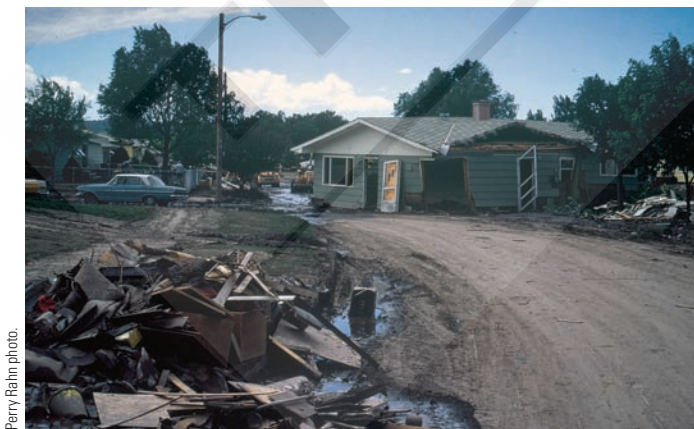
▶ FIGURE 12-28. This house was carried off its foundation onto the road by the 1972 Rapid City flood.
