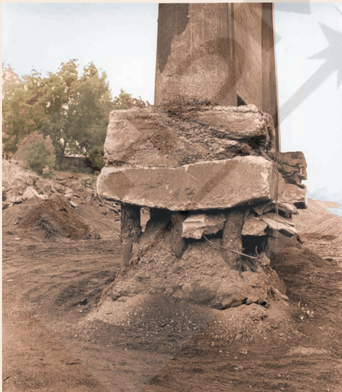
▶ FIGURE 12-40. Dry Creek bridge supports near Healdsburg, California, have been severely undercut by stream-bed gravel mining downstream.
