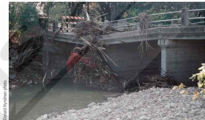
► FIGURE 12-42. A catastrophic flood on this small stream, Shoal Creek, in Austin, Texas, on November 15, 2001, overtopped the bridge deck and left branches tangled in its railings, evidence of the previous flood height. The high water also deeply eroded the channel and undercut the supports, causing the bridge deck to sag.
