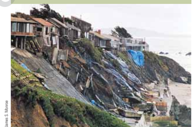
► Figure NC.62 Mass wasting in Bodega Bay resulted from undercutting of the sea cliff by waves generated during winter storms of 1997–1998.
